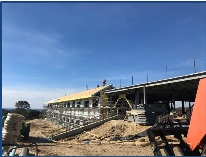
San Dieguito High School Academy Arts & Humanities Building
